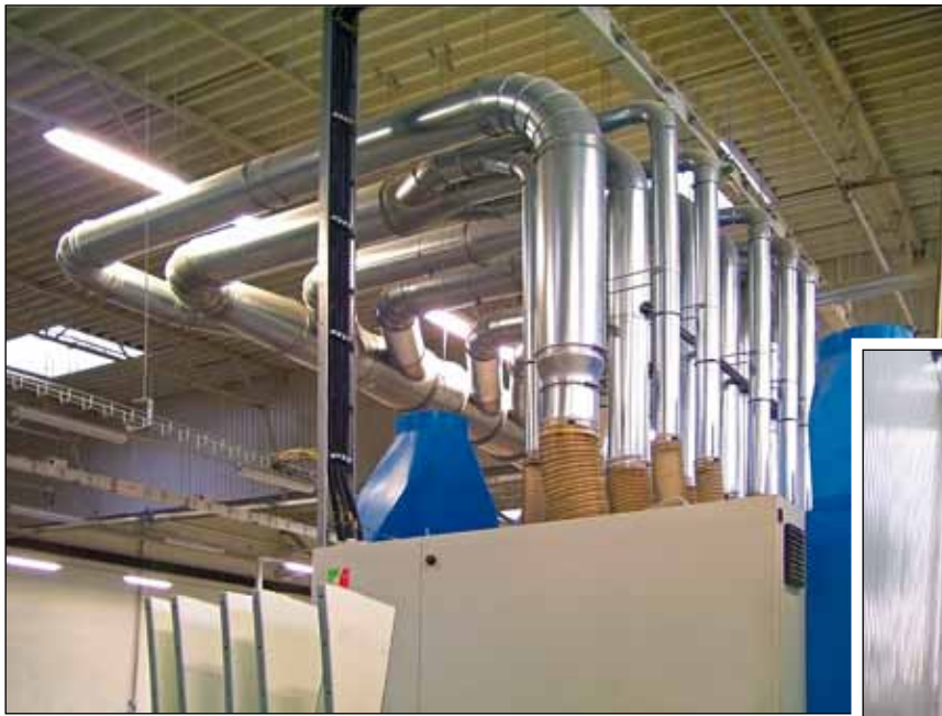
Agaard chain filter at Danish pinewood furniture factory - air volume: 120,000 m 3 /h.
