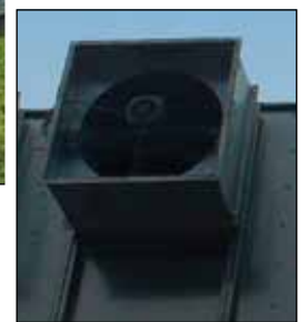
Close-up of Aagaard sound insulated reverse-air fan.
